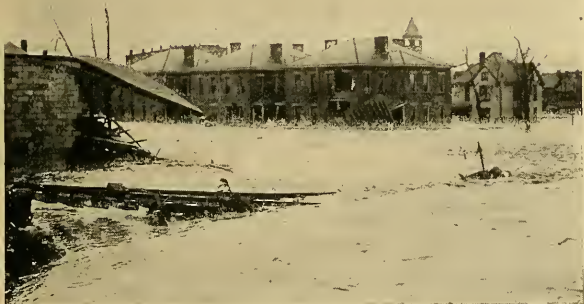
COLUMBUS: BRICK HOUSES BATTERED BY HEAVY DRIFTWOOD
